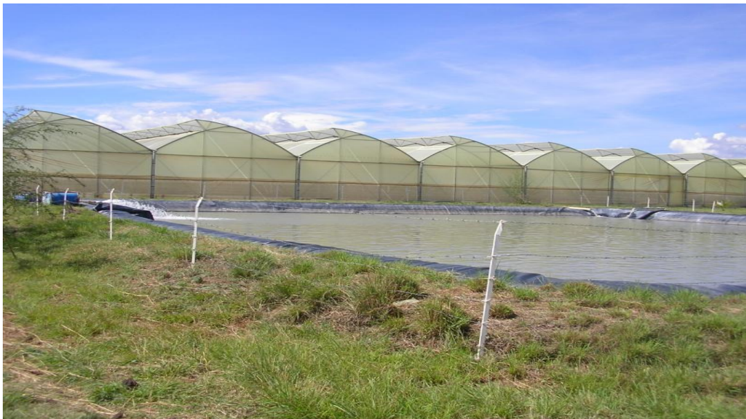
Figure 9.2: Water Reservoir in Sebeta
