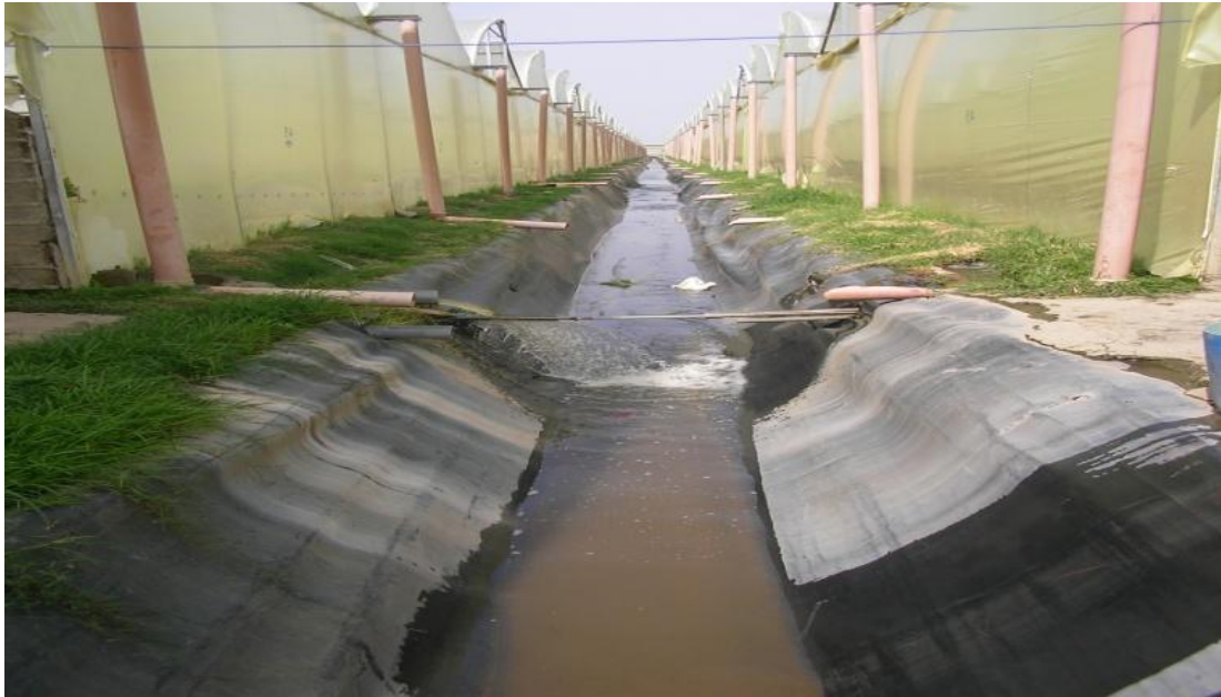
Figure 9.5: Drainage Channelled to Lake Zeway
