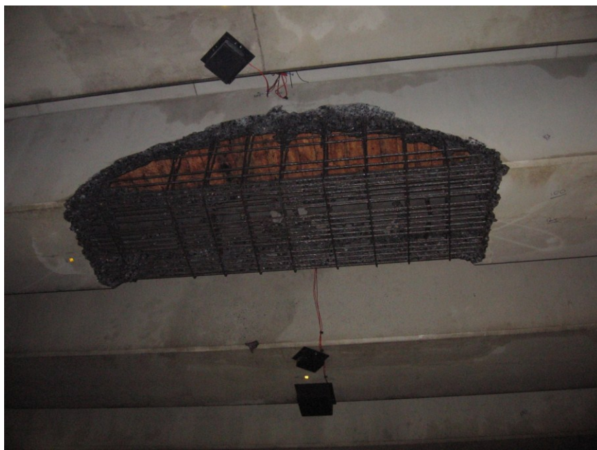
Figure 5 – Removal of Concrete through Hydrodemolition
