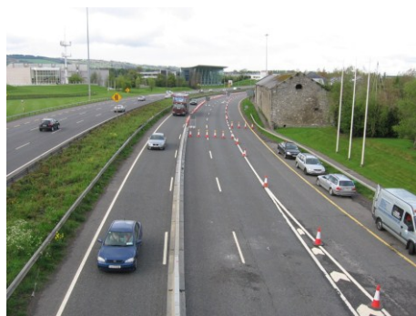
Figure 8 – Traffic Management Provided during Rehabilitation
