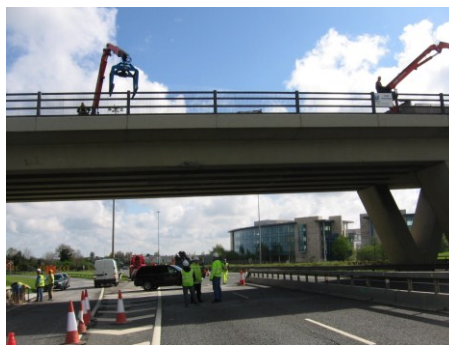
Figure 7 – Removal of Preload
