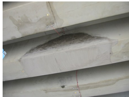
Figure 6 – Repaired Section of Damaged Beam
